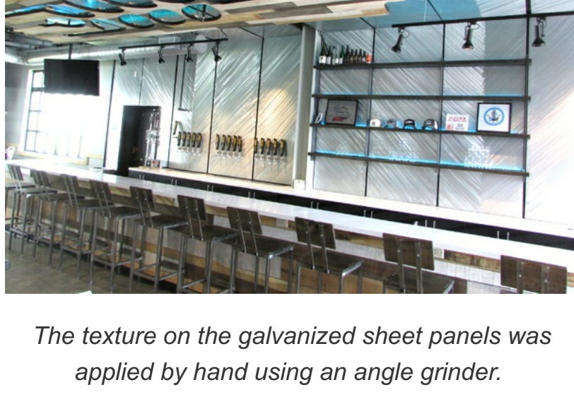
The texture on the galvanized sheet panels was applied by hand using an angle grinder.
